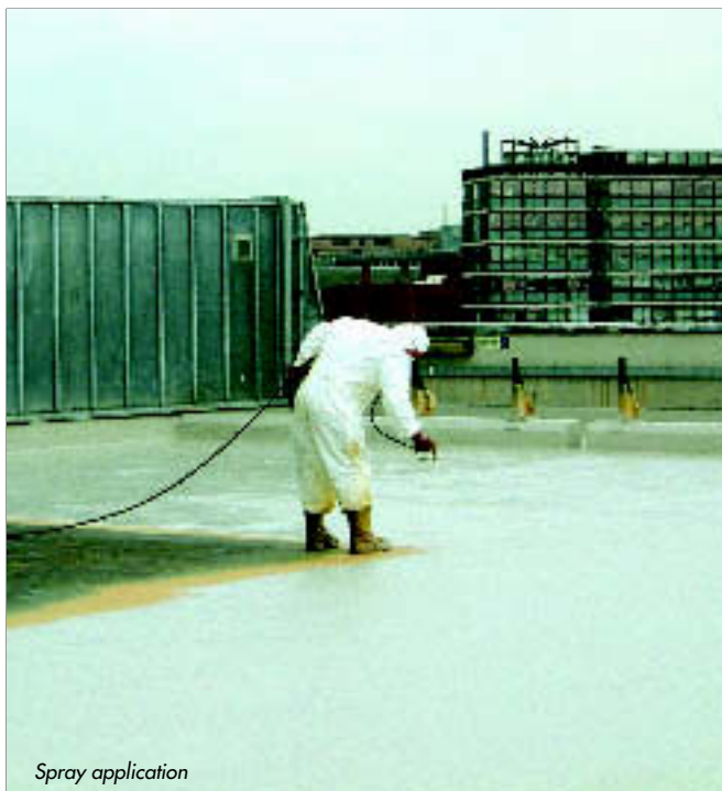
Inverted warm roof application
